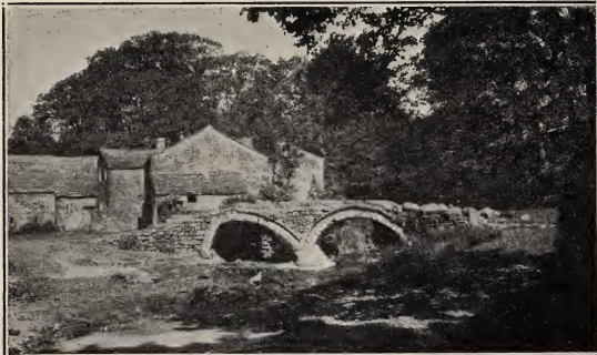
Bridges interest the missionary. Rock and slate are the chief materials used in the construction of country buildings and bridges.
