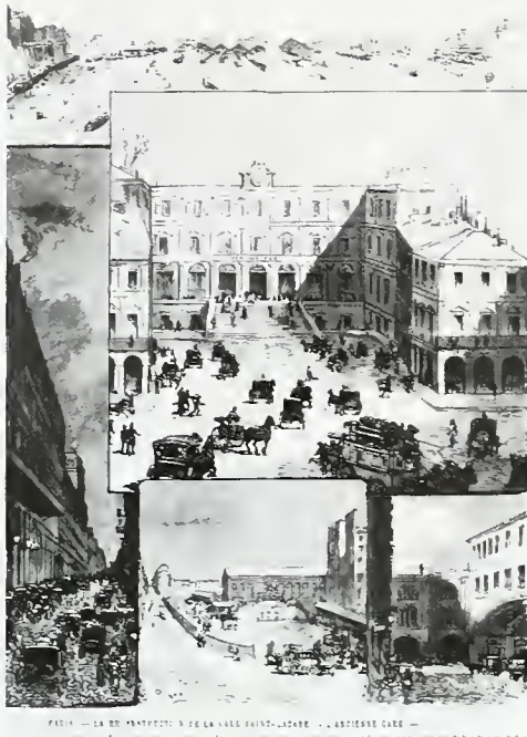
Fig. 29. Paris— The Rebuilding of the Gare Saint-Lazare—The Old Station (1. View from the Pont de l'Europe.—2. Main station entrance.—3. Entrance to the main lines, rue d'Amsterdam.—4. The exit yard and the wooden bridge of the rue de Rome.—5. The Cour Bony.), 1885. Photo: La Vie du Rail, Paris.
