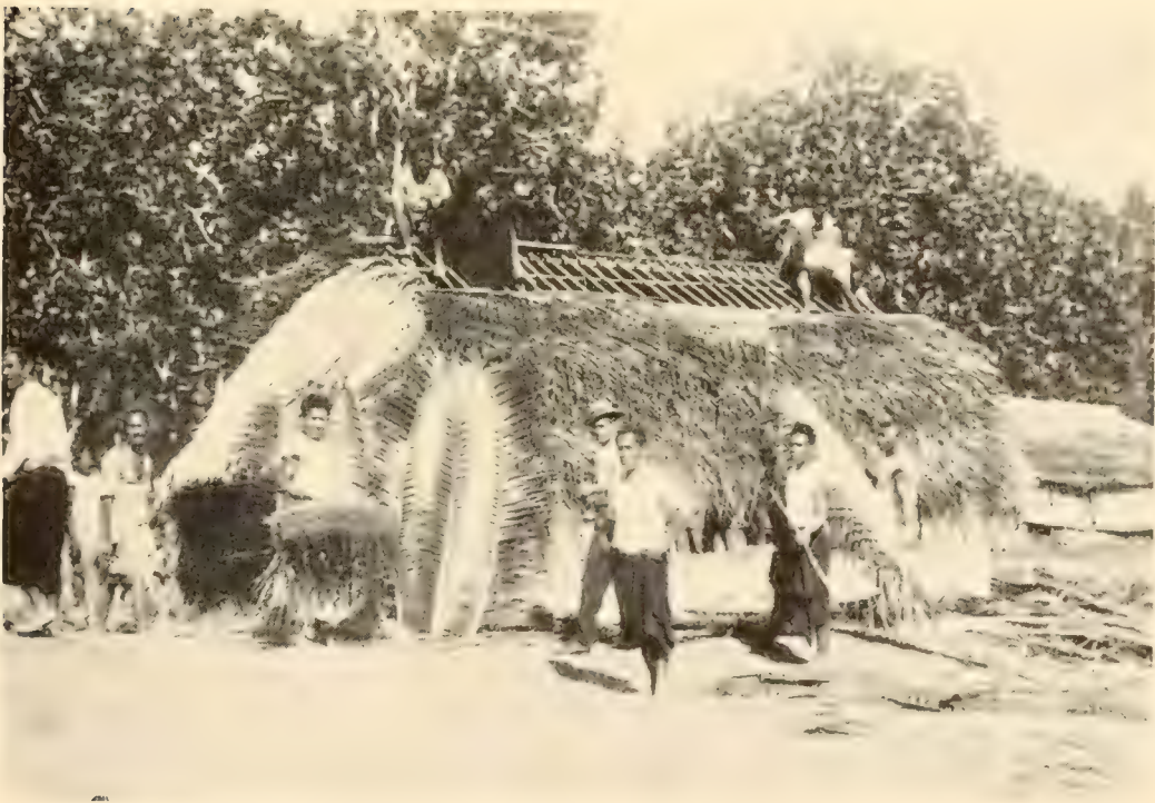
FIG. 68.—Natives roofing a house with the fronds of the cocoanut palm. Very little sugar cane, the leaves of which are generally used by the South Sea Islanders as thatch, is grown on Niaufoou. (Photograph by Kellers.)
