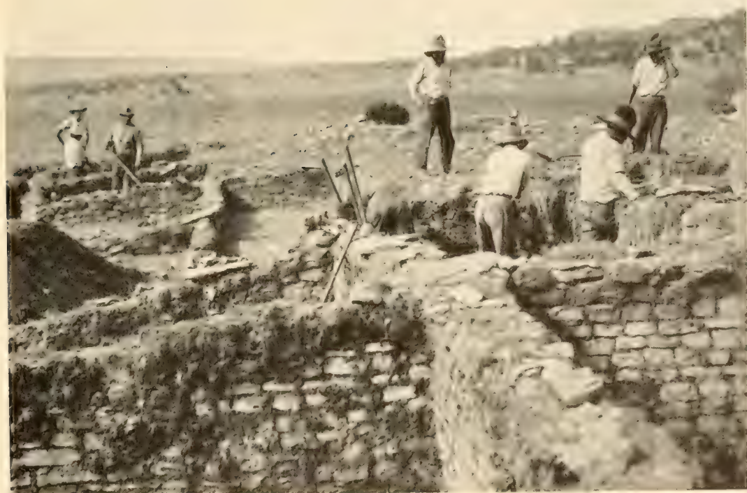
FIG. 160.—Removing débris from the small house.
