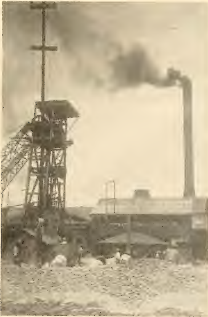
FIG. 31.—Patio of the Santa Maria de la Paz mine with workmen breaking ore by hand.
