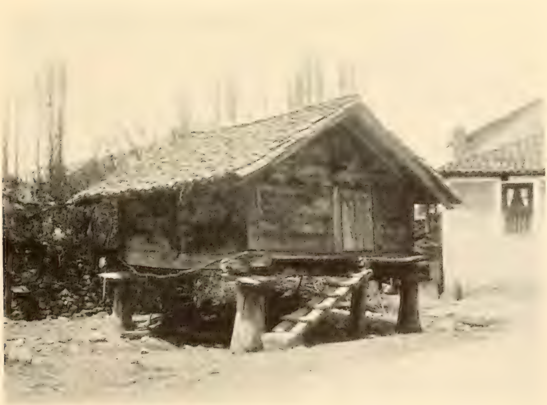
FIG. 46.—A storehouse for grain in Riaño. Note the flat stones at the corners to prevent entry of rats.
