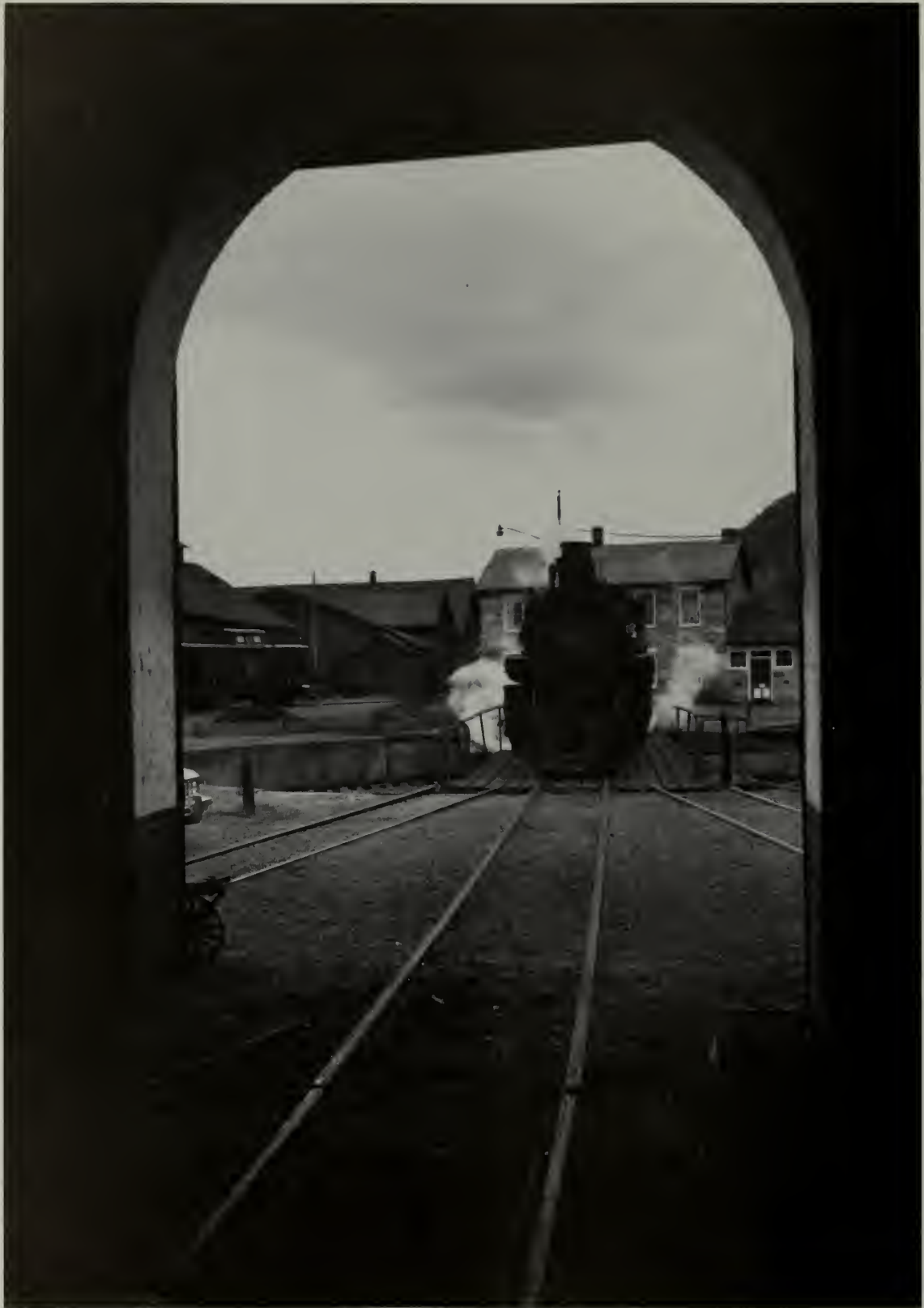
FRAMED BY THE ARCHED PORTAL TO A STALL IN THE BRICK ROUNDHOUSE, EBT'S #15 SITS ON THE TURNTABLE BRIDGE IN THE RAILROAD YARD AT ROCKHILL. To the left of #15 is one of the two eight-wheel cabooses and a portion of the shop complex. Directly behind #15 is the late 18th century farmhouse, which was on the farm property that the EBT purchased in the 1870s for its main yard and shop complex site.
