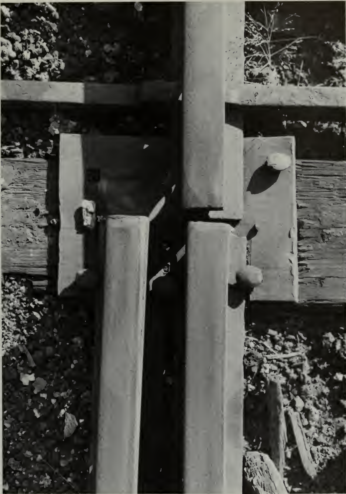
MANY STUB SWITCHES REMAIN IN USE IN THE EBT'S YARD. An 18th century standard, these were replaced in later years on main line EBT tracks by blade switches, which are universally used today. This photo looks directly down on the point where the single track coming from the top of the picture divides into two tracks. The top rail is embraced in an iron bridle just above the wooden crossie. The bridle connects to a vertical lever on the switchstand adjacent to the track. By heaving on the lever, the railroad crew can move the top rail's alignment from one to the other of the lower rails.
