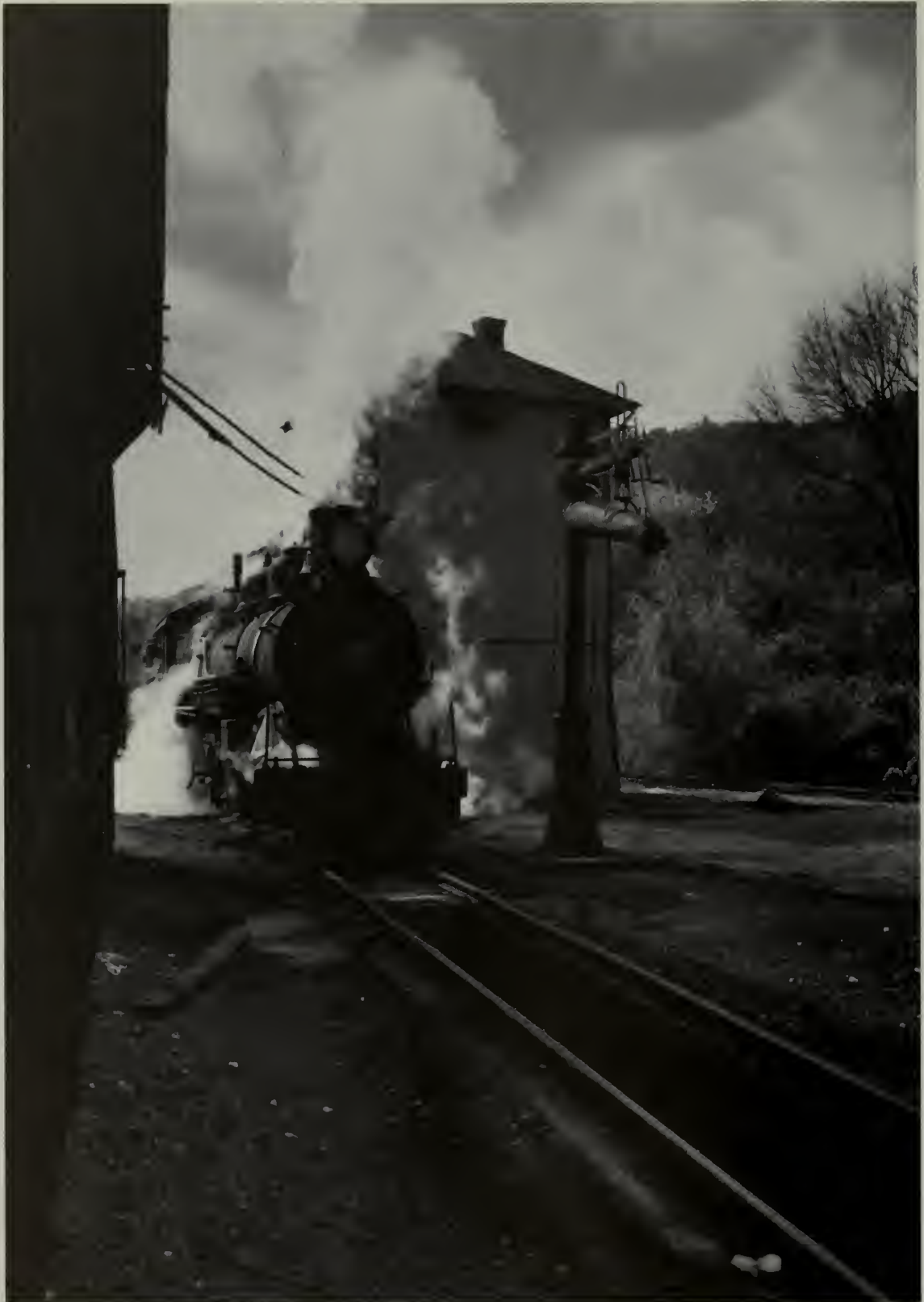
LOCOMOTIVE #15 ON THE LEAD TRACK TO THE ROUNDHOUSE IN ROCKHILL. The back wall of the railroad's boiler shop is on the left. A concrete inspection pit is between the rails in the foreground. Beside #15 is one of three water columns in the yard, which were used to water the locomotives. The columns were gravity-fed from a reservoir southeast of the yard.
