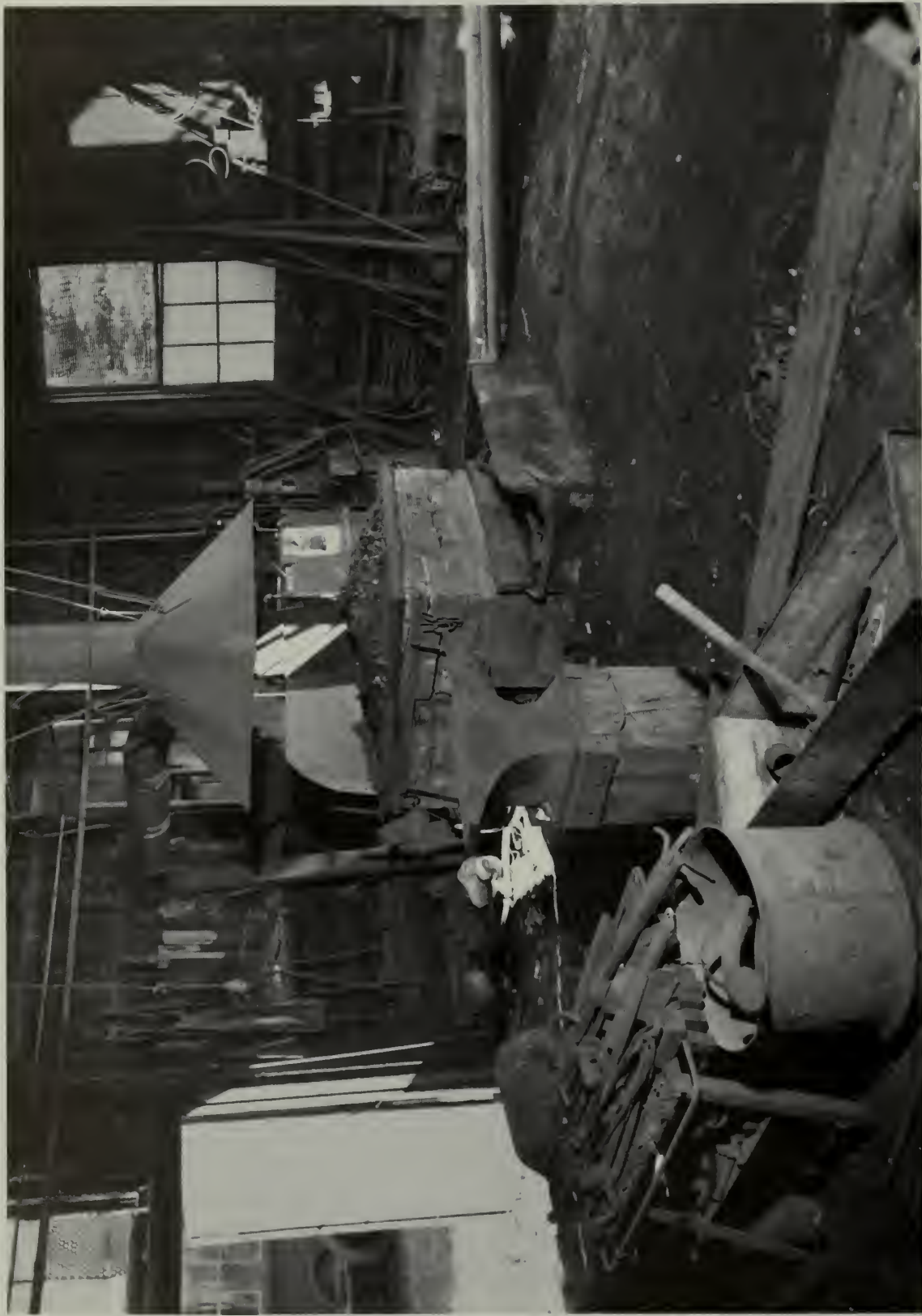
THE FORGE AND MASSIVE ANVIL IN THE EBT'S BLACKSMITH SHOP. Almost all of the tools used in the EBT shops were made on site, many starting here, beaten and bent into shape by hand.
