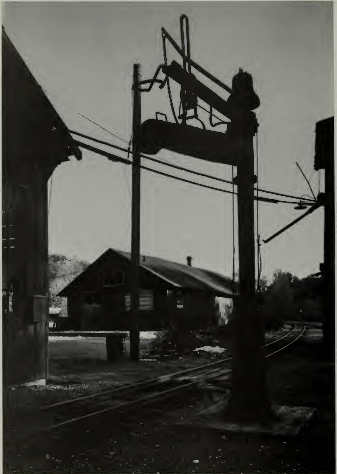
A WATER COLUMN ON THE LEAD TRACK TO THE EBT ROUNDHOUSE IN ROCKHILL. A corner of the boiler shop is on the left, and behind the column is the carpenter shop. The water column would swing over the track 90 degrees to line up with the tender's water hatch.
