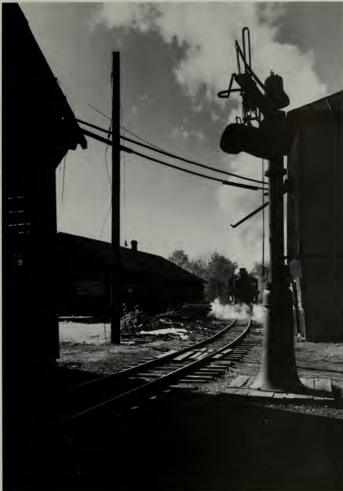
NUMBER 17 BACKS AWAY FROM THE ROUNDHOUSE TOWARD THE COALING DOCK AT THE SOUTH END OF THE YARD COMPLEX. In silhouette is the thin pipe used to deliver specially dried fine sand from the sand house, which is in the right of the photograph. To get sand, a fireman would stand on the locomotive's running board and pull a chain; releasing the chain would stop the flow. The insulated pipes running across the track carried steam from the boiler shop to the sand house, which was essential for heating the sand and keeping it dry and loose. The dry sand was used for added traction on grades and starting on slippery rails.
