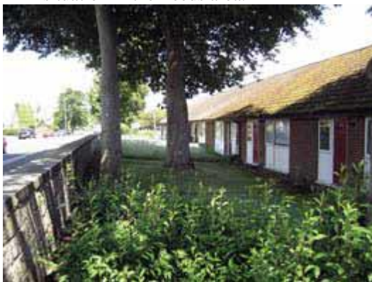
Poor relationship: Beech trees at 4m from the front of a dwelling are overbearing and cut out light.
